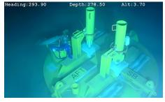
**Mooring lines support for offshore windmills /** Seabed securement via suction anchors
